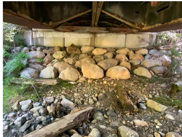
Right Bank Abutment when facing downstream
