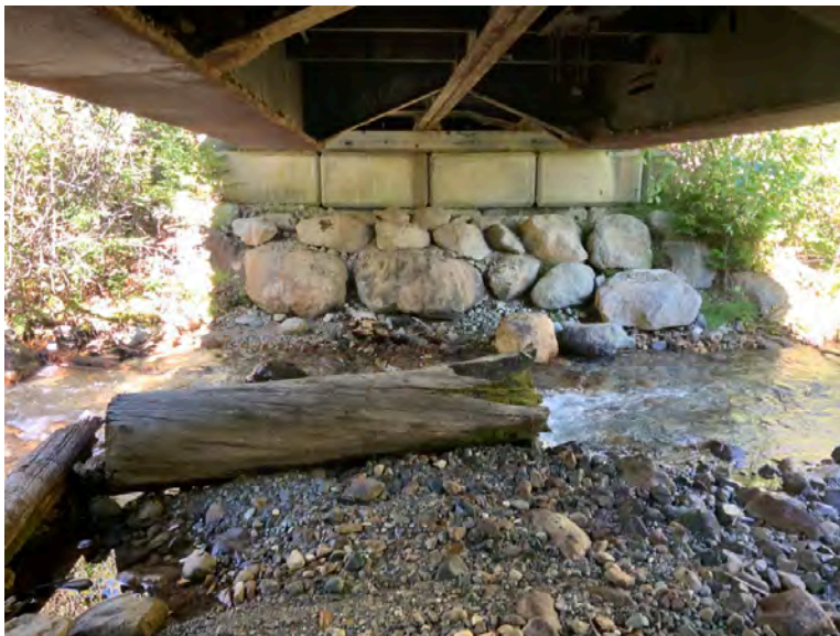
Left Bank Abutment when facing downstream
